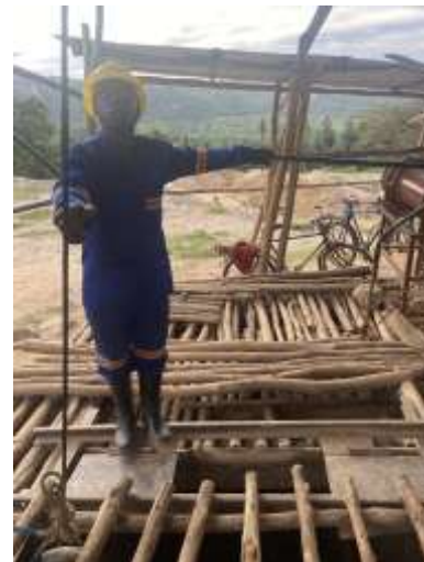
Pulley for delivery material
