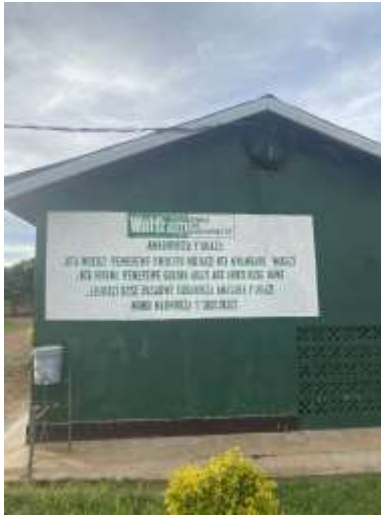
WMP upgrading plant
